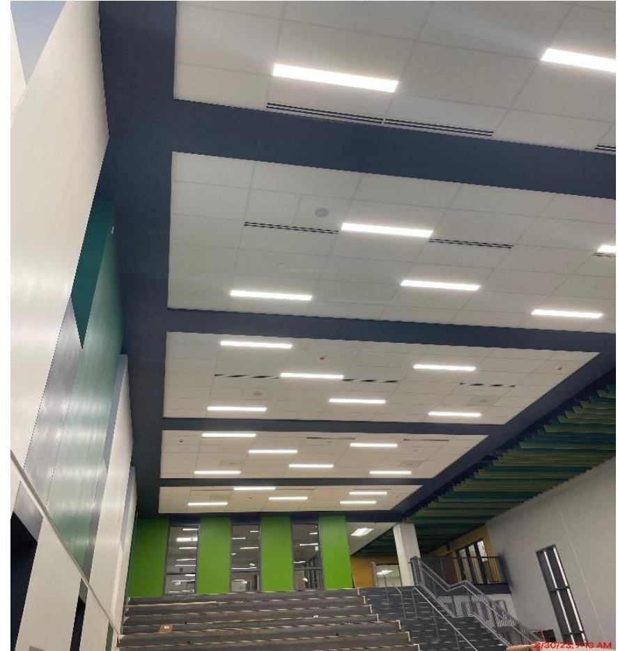
Ceiling at the Learning Stairs - West Wing
