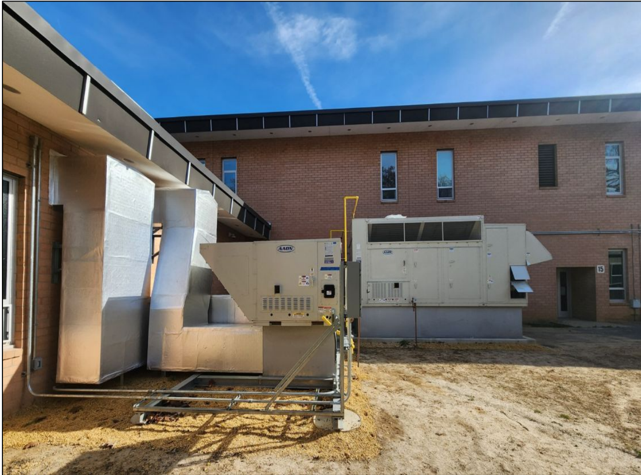
RTU #3 and DOAS #1 Installed & Started Up
