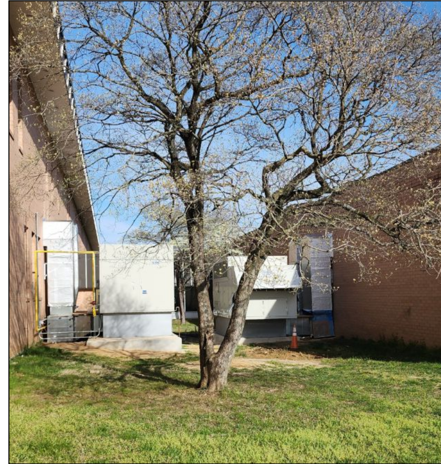
DOAS #2 and RTU #1 Installed & Started Up
