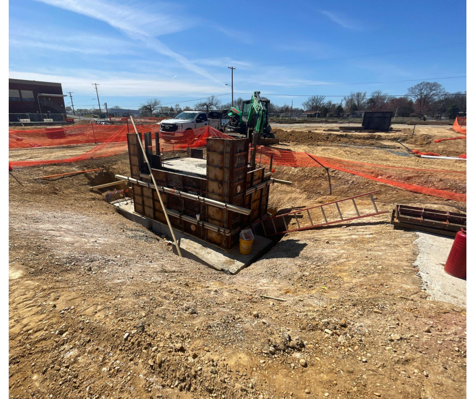
Elevator Pit and Stair 2 Footing
