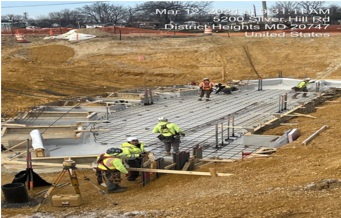
Foundation - Orchestra Mud Slab Foundation Orchestra Pit
