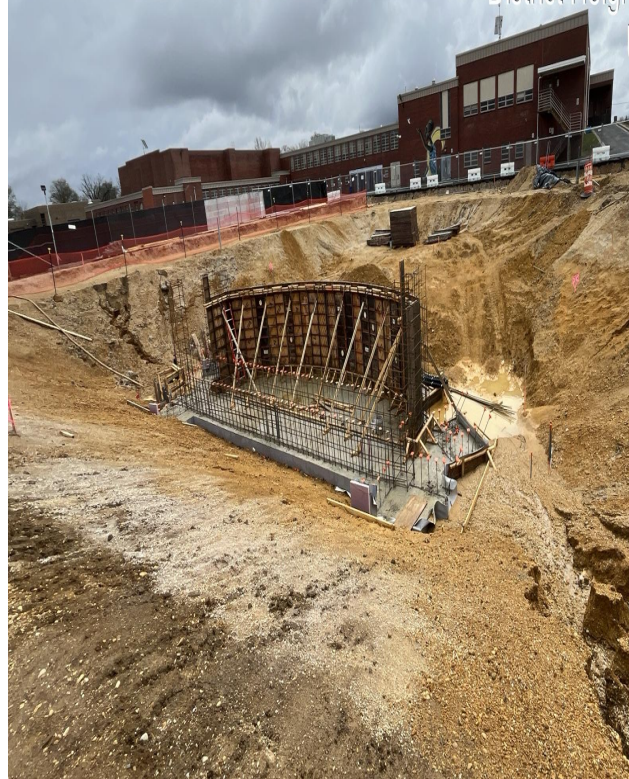
Foundation Orchestra Pit Wall Framing
