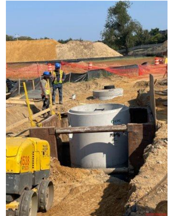
Installation of the middle base of manhole (MH) 96
