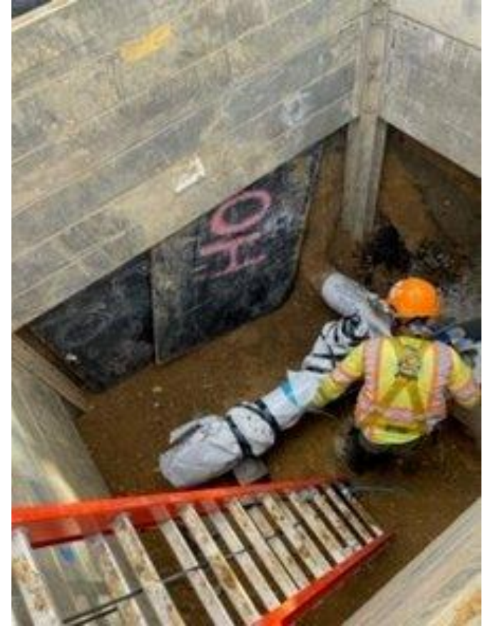
Water line tie-in to existing
