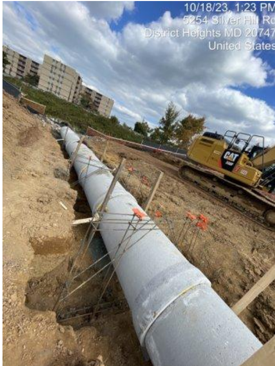
Installation of storm piping from RS-2 to I-149
