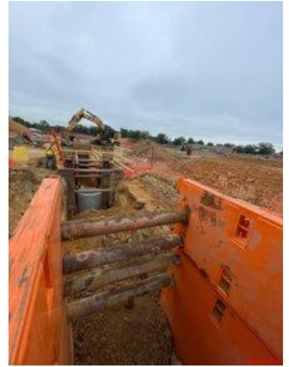
Excavation work near MH 3.
