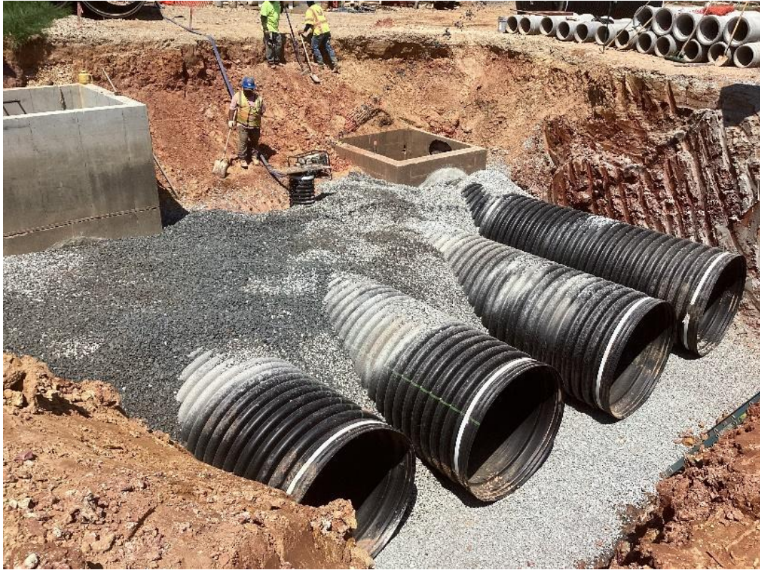
Stormwater Ground Work
