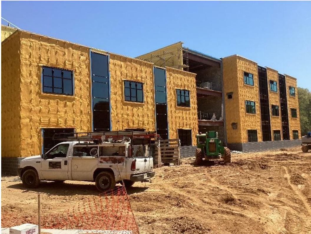
Area B & C – Spray Foam, Curtain Walls, Windows
