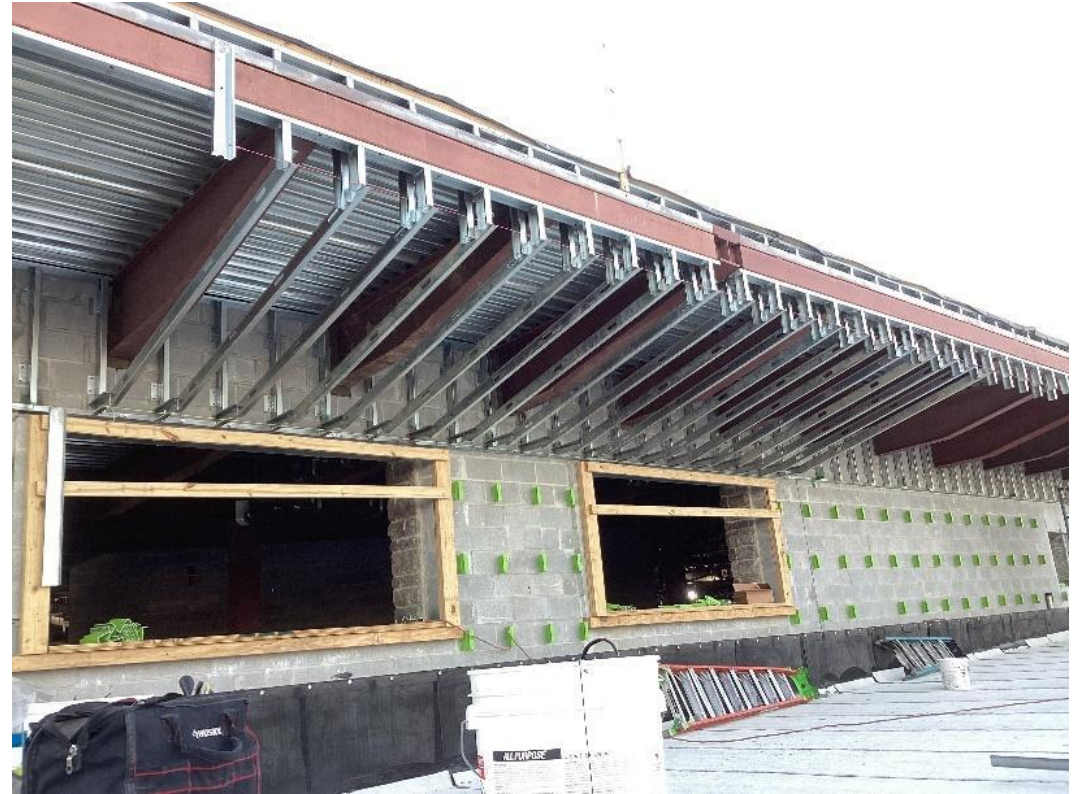
Metal Soffit Framing
