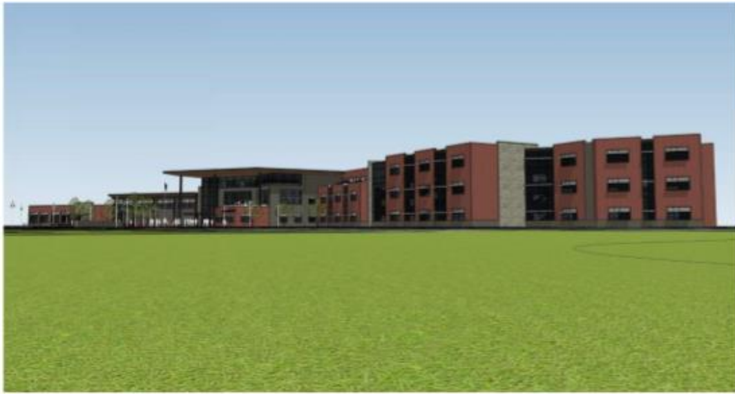
MAIN ENTRY / CLASSROOM WING - VIEW FROM SOUTHEAST
